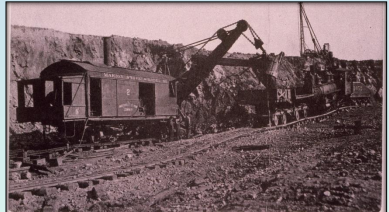
Figure 45: Iron Mining in Progress at the Open Pit MAYVILLE MINE - Circa 1911 This large steam shovel, belonging to NORTHWESTERN IRON CO., was a Marion Shovel - Model 60 , built by the Marion Steam Shovel Co., of Marion, Ohio. A steam-powered drilling rig, used for exploratory test-drilling, can be seen standing on top of the ledge, above the ore train.
