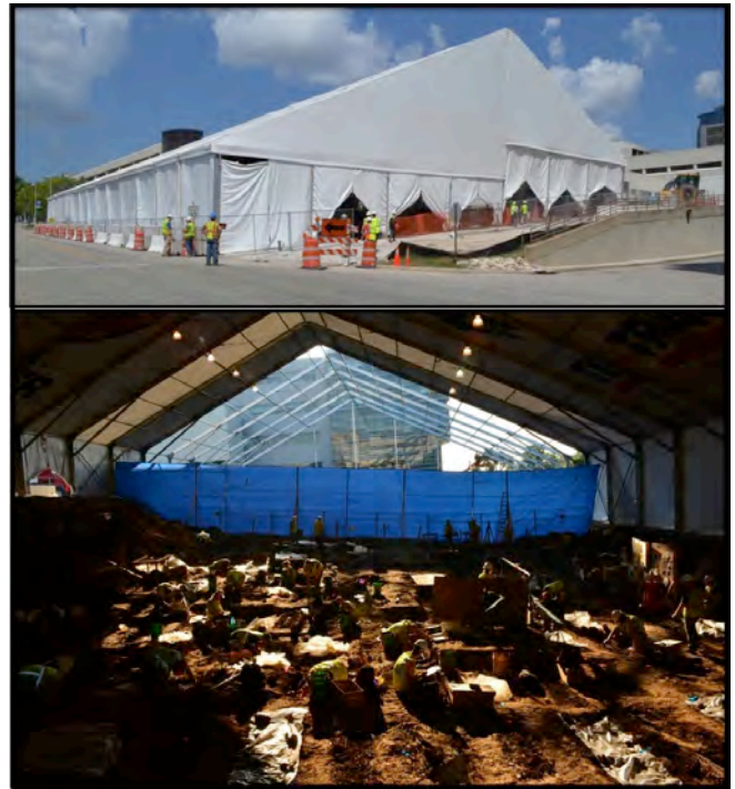
Figure 4.6. Exterior and interior of the excavation tent (UWM photo on file, UWM-ARL).
