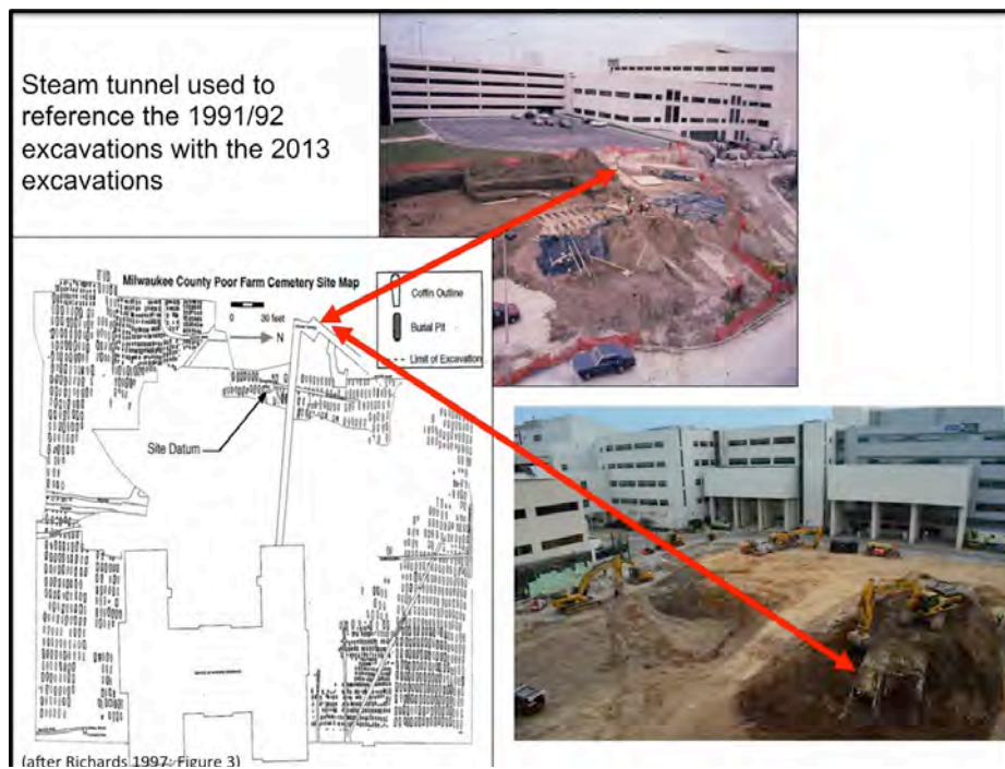
Figure 4.36. Overview of the steam tunnel used to reference the 1991-1992 excavations with the 2013 excavations (GLARC and UWM photos on file, UWM-ARL).
