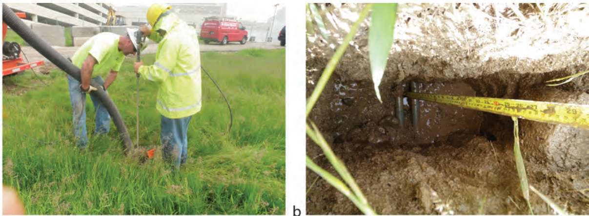
Figure 4.39. Ground hydro-vacating within the boundaries of Cemetery 2 on May 29, 2013 (UWM photo on file, UWM-ARL).
