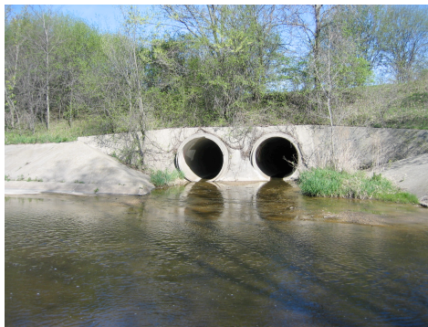
Figure 2: Example of Stormwater Outfalls.
