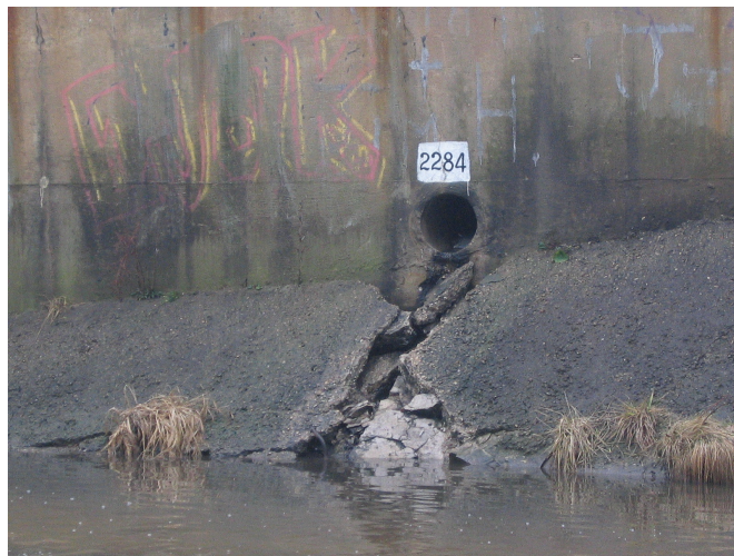
Figure 2. Stormwater outfall on Honey Creek.
