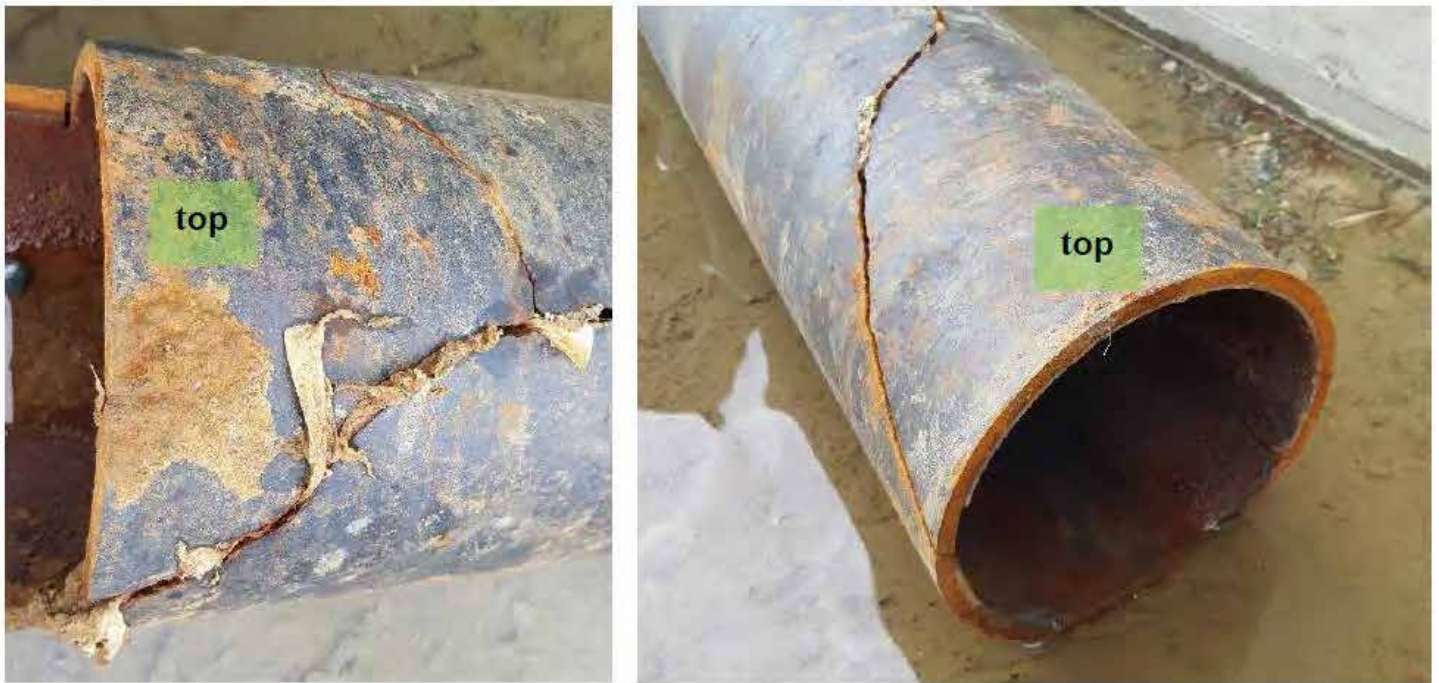
Figure 9: Wayne Creek watershed site map used for assisting in location of contamination sources – photographs of the resulting identified cracked pipe as the source.
