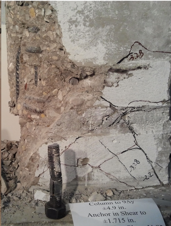
S2 (cyclic shear along with cyclic column deformation)
