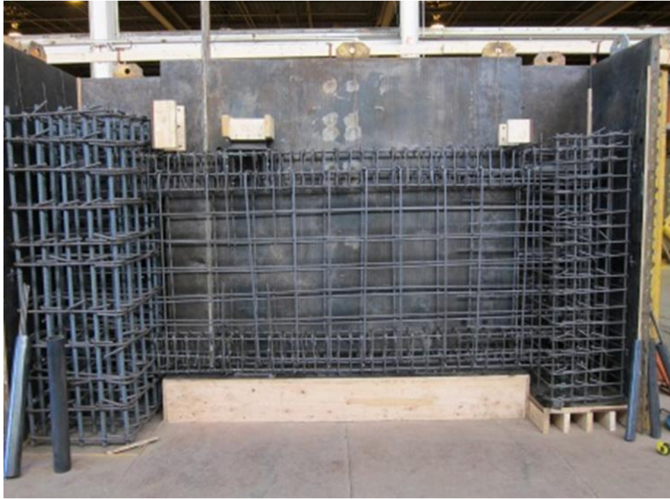
Figure C.8: Photo of Wall Specimen Right Before Concrete Placement
