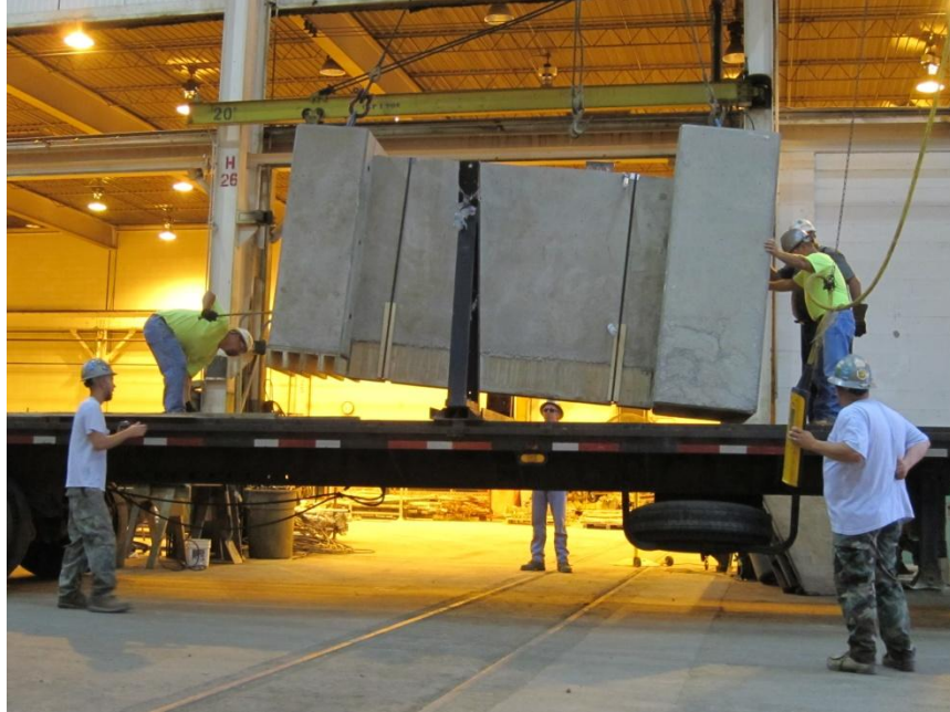
Figure C.14: Photo of Wall Specimen to be Transported to UIUC
