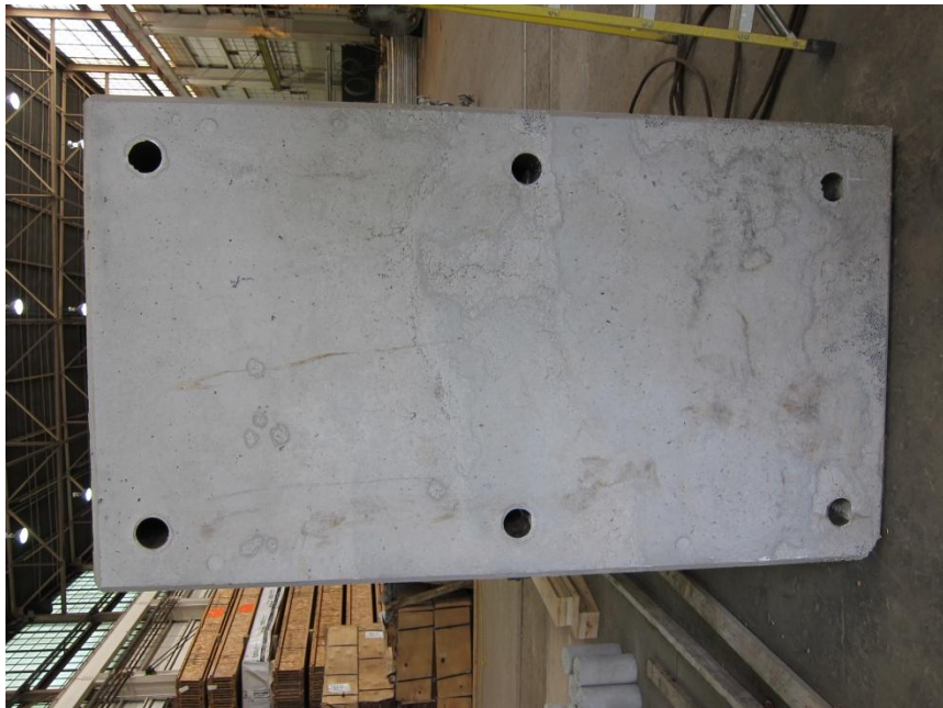
Figure C.15: Photo of Wall Footing and Floor Post-tensioning Holes
