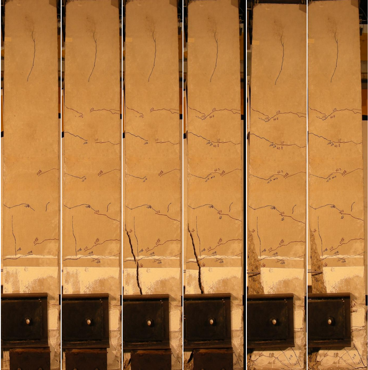
(a) \pm 0.58 in. (b) \pm 1.12 in. (c) \pm 1.66 in. (d) \pm 2.20 in. (e) \pm 3.28 in. (f) \pm 4.9 in. Figure A.28-Crack map of S2 under various loading cycles
