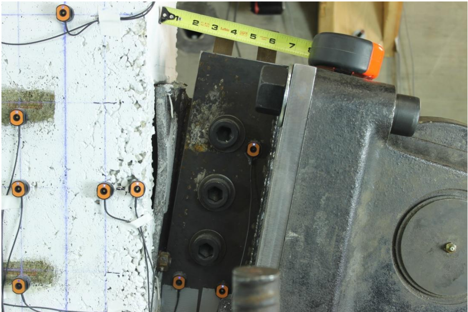
Figure 5.12: Photo of right anchor connection at failure
