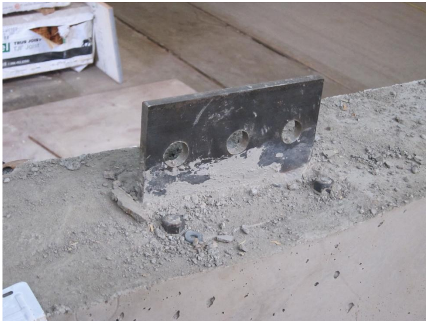
Figure C.13: Photo of Shear Tab
