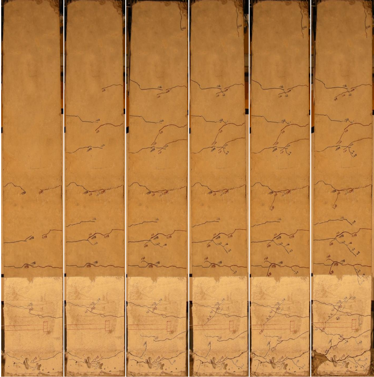
(a) \pm 0.58 in. (b) \pm 1.12 in. (c) \pm 1.66 in. (d) \pm 2.20 in. (e) \pm 3.28 in. (f) \pm 4.9 in. Figure A.14-Crack map under various loading cycles (T3)
