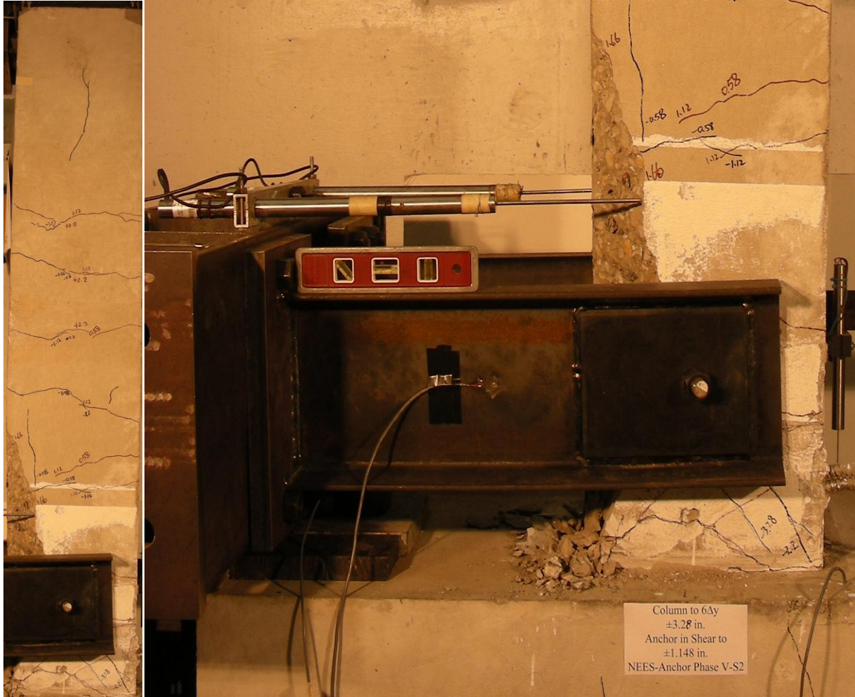
(a) Column crack pattern
