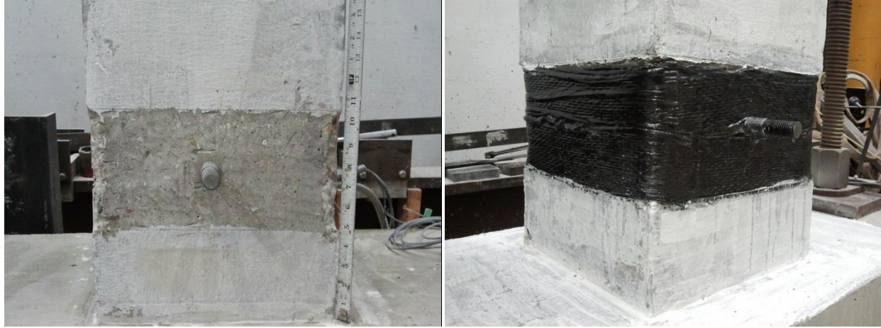
Figure 4.32: FRP wrapping of Specimen S3
