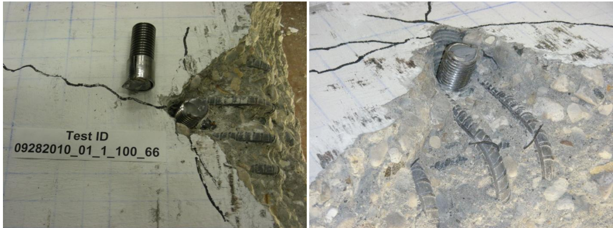
Figure 5.4: Concrete cover pushed off during shear tests of 1.0-in. anchors
