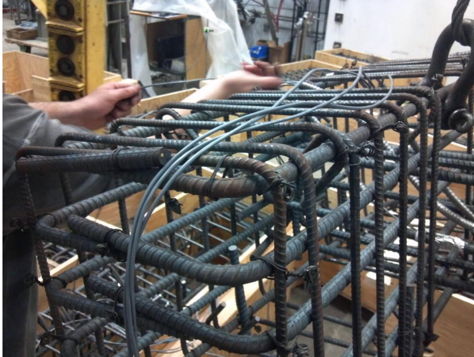
Figure 4.13: Surface reinforcement in the tension tests of reinforced anchors
