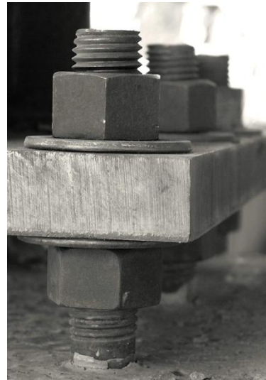
(b) anchors without grout
