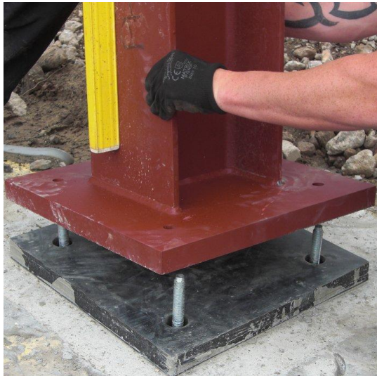
(a) anchors with leveling grout
