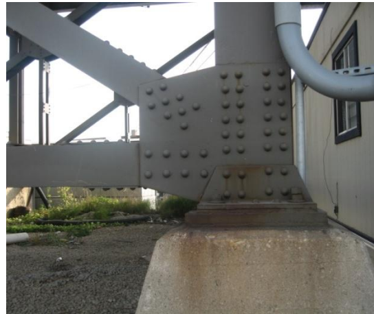
Figure 1.1: Typical anchor connections between structural steel and concrete
