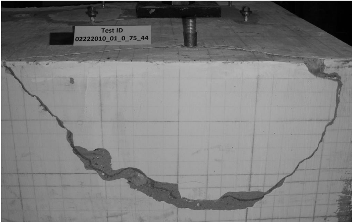
Figure 1.4: Concrete breakout failure in shear
