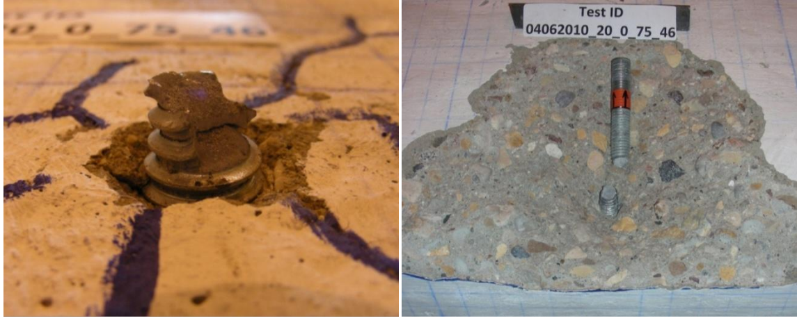
Figure 4.14: Concrete spalling during tensile steel failure
