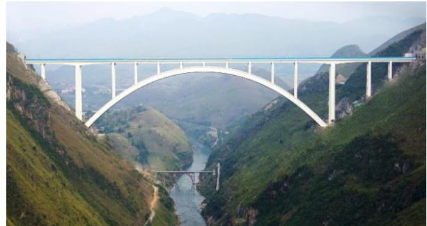
Fig. 2 – Beipanjiang Railway Bridge
