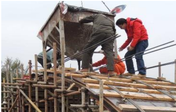
(a) Under construction
