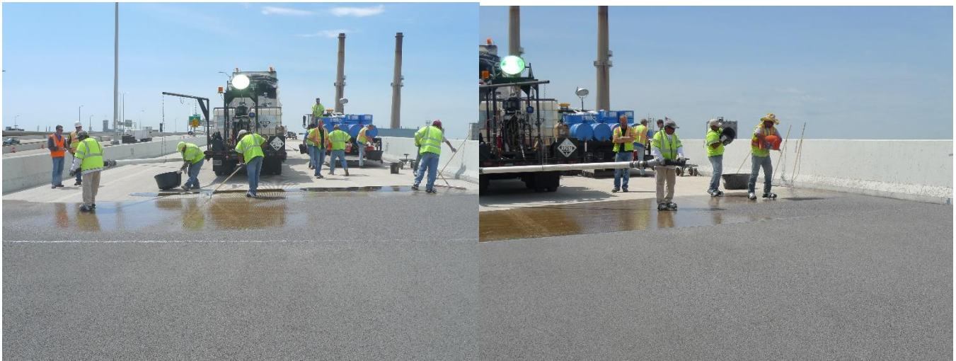
Figure 30. Placement of resin and aggregate on a 2-lift overlay system.
