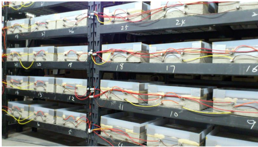
Figure 3. Group B and C specimens undergoing initial chloride/accelerated corrosion exposure.
