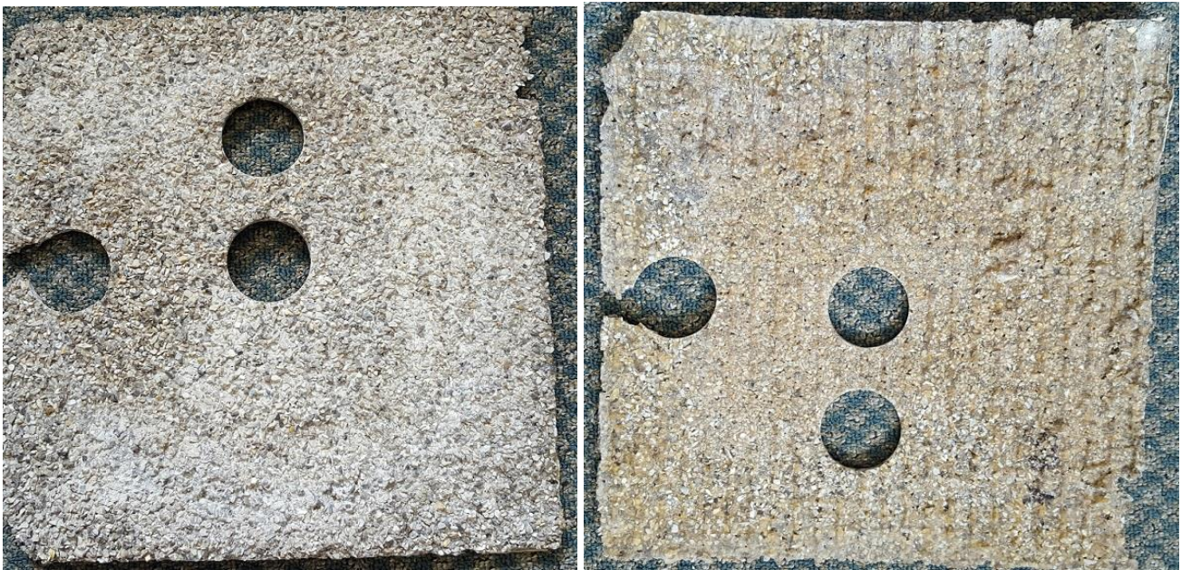
Figure 39. Pictures of delaminated overlay from a S8 specimen: top surface (left), bottom surface (right).
