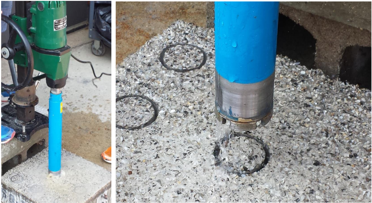
Figure 23. Coring drill setup.
